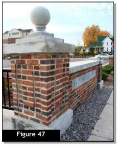
The above structural screen utilizes masonry columns and fencing to provide a visual and physical buffer between a sidewalk and parking area.
