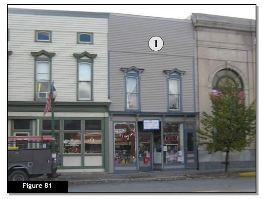
The use of inappropriate materials and finishes (1) diminishes the visual quality of the structure and adjacent buildings. In this example, although the structure has a high quality storefront, the use of vinyl siding over what was likely masonry construction reduces the overall appeal of the building.
