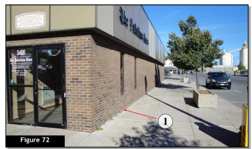
The building façade shall not abruptly end at the sidewalk (1). The building shall have a base of material that anchors the structure to the site  $[\S 112-17G(2)(a)]$
