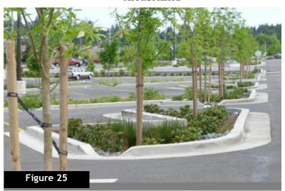
Where appropriate, bioretention aeras and bioswales similar to the above may be used to promote the infiltration of storm water. These installations would be appropriate in parking lot medians or in linear strips along drive aisles or behind parking lots in lieu of large, unsightly retention facilities
