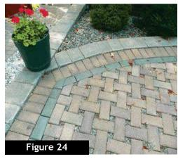
Porous pavements are encouraged to further facilitate infiltration and slow storm water runoff. These materials are especially useful along the periphery of parking areas and/or adjacent to bioretention areas (below).
